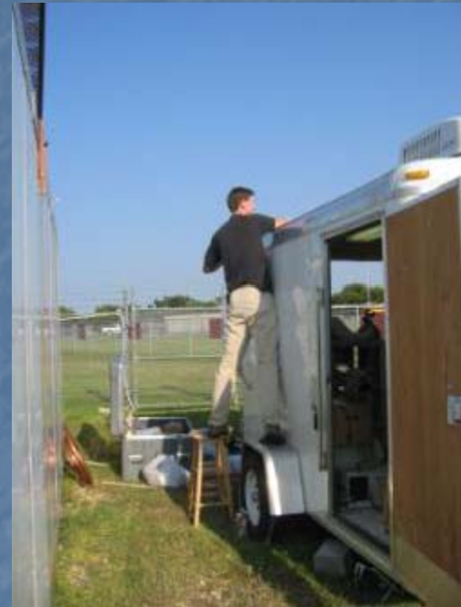
Inlet Installation, Deer Park Site
