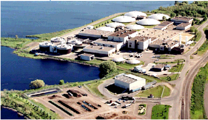
Western Lake Superior District wastewater treatment plant in Duluth, MN
