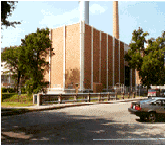
Figure 1. UT Austin's CHP Facility. Source: UT Austin.
