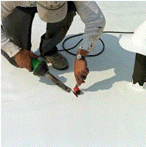
Installing highly reflective roofing in Atlanta
